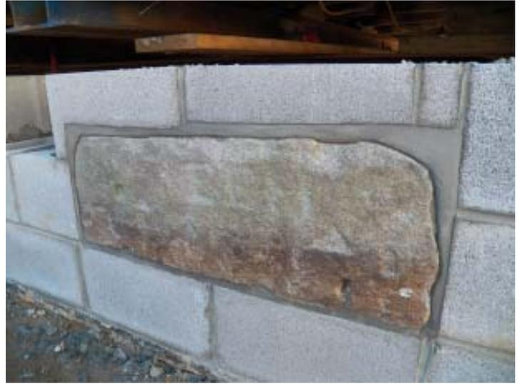
The Schoolhouse stands on I-Beams above the foundation. The blocks have been installed with gaps to allow for the I-beams to be removed and the building lowered onto the foundation. Masonry work and excavation was done by Sinopoli Contractors, Inc., of Hawley Rd., Oxford.
